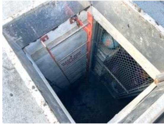
Reinforced concrete roof deck.
