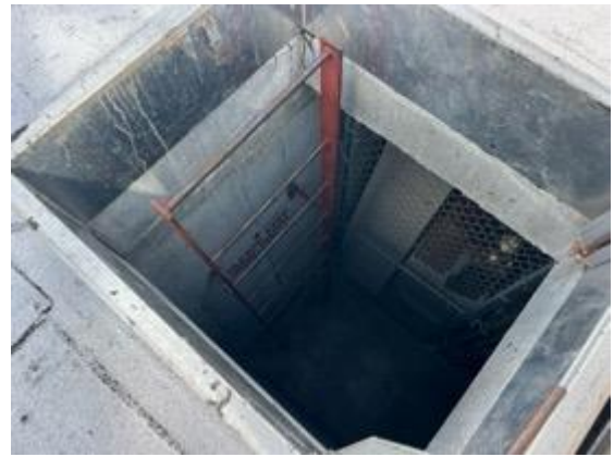
Reinforced concrete roof deck.
