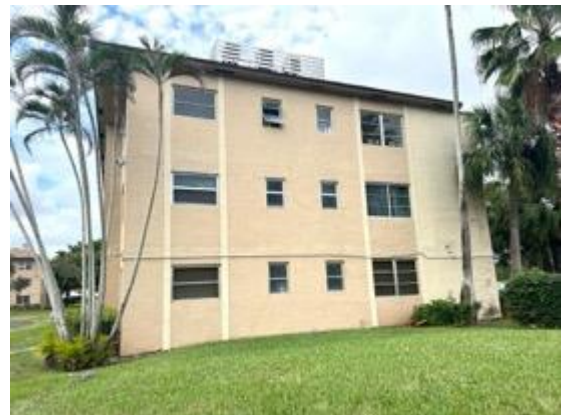
Building left side view.
