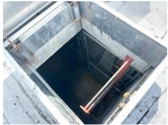
Reinforced concrete roof deck.
