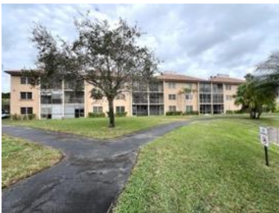
Building rear view.
