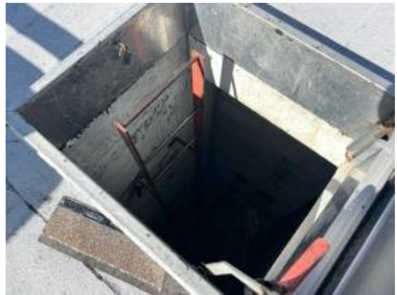
Reinforced concrete roof deck.
