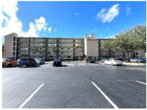
Building front view.
