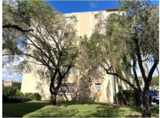
Building left side view.
