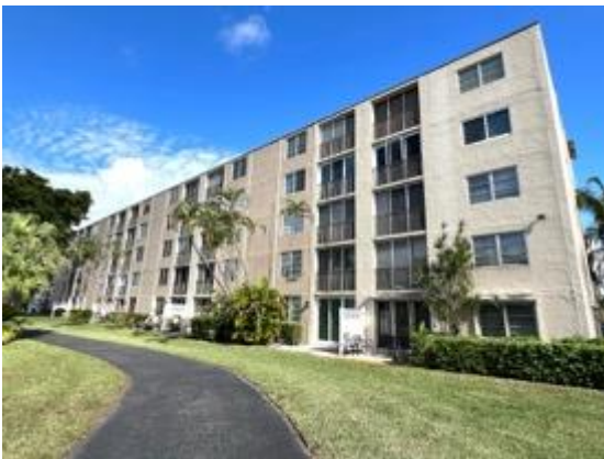
Building rear view.
